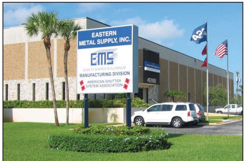
The ASSA World Headquarters and EMS Shutter/Manufacturing Division are located in West Palm Beach, Florida
